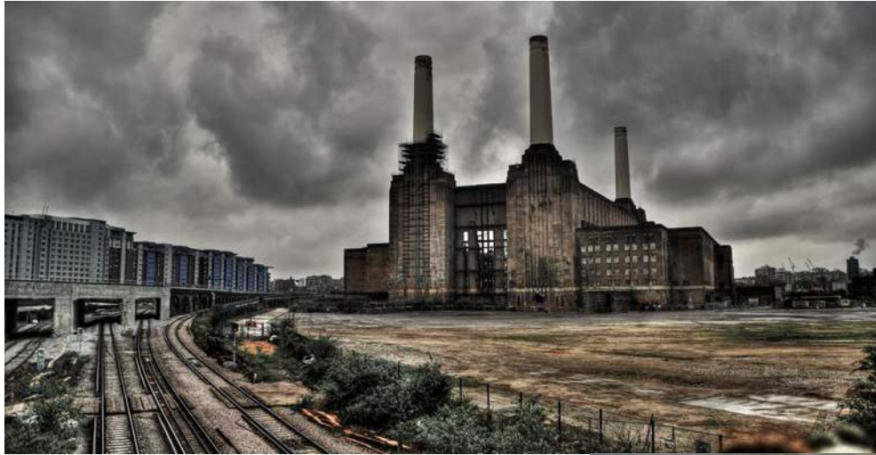
A closed power station
