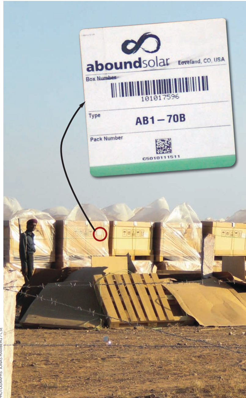
Rajasthan imports modules from the US for a project under JNNSM
